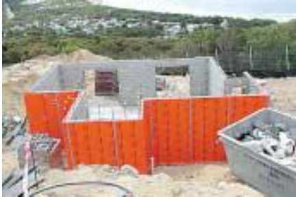
Photo 1 Kordon TB - full retaining wall
