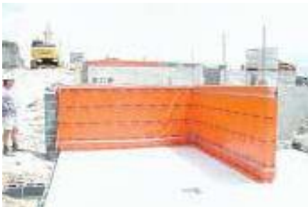
Photo 3 Kordon TB - internal wall treated
