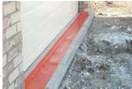
photo 1 garage entry detail secured with the aid of 3M "super 77" spray or similar Note: where various slab conditions prevail i.e. rough or damaged:- It is important to establish a full seal to the perimeter is achieved
