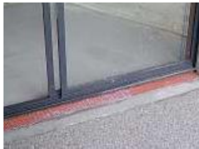
2. renderlok secured to masonry with approved concrete nails. - (15mm length preferred)
