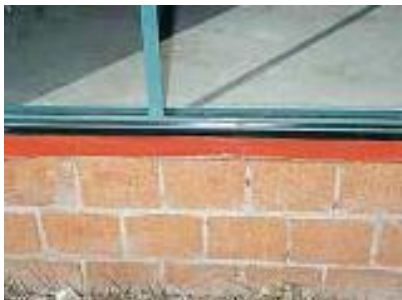
2. renderlok secured to masonry with approved concrete nails. - (15mm length preferred)
