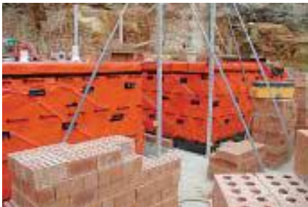
Photo 2 Kordon TB - retaining/stepdown
