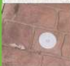
Installation through concrete.
