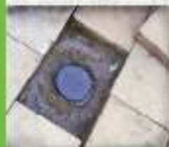
Installation under pavers.
